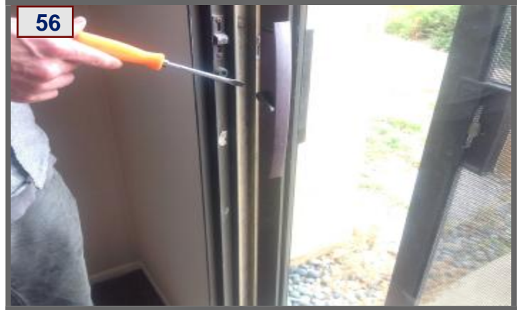
Master Bedroom Sliding Glass Door Will Not Lock Hard to Open or Close
