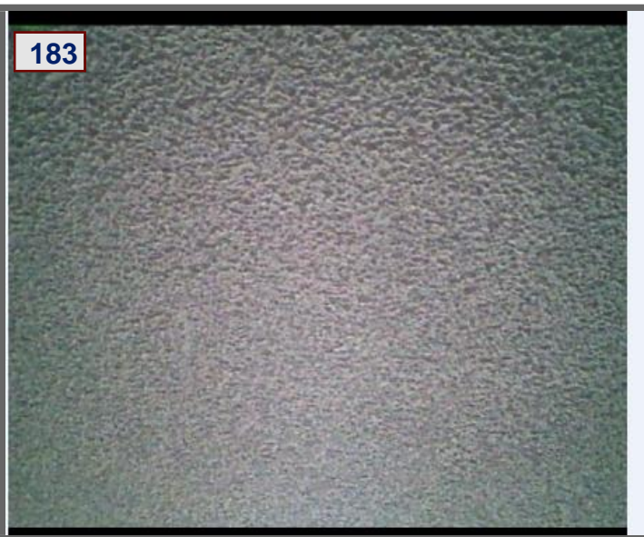
Ceiling Repaired in Bedroom 1 No Moisture Noted
