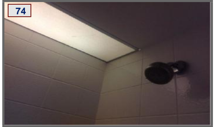
Master Bath Electric Light Not In Code
