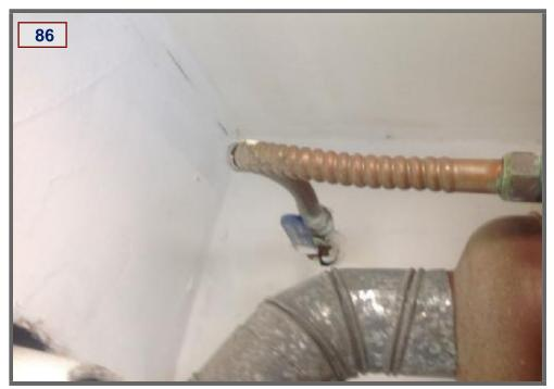
Hot Water Heater Shut off Valve Corroded
