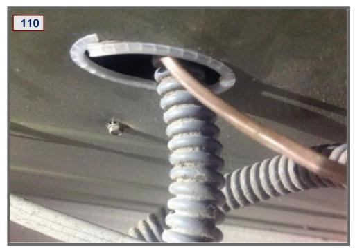
Gas Line In Properly Installed
