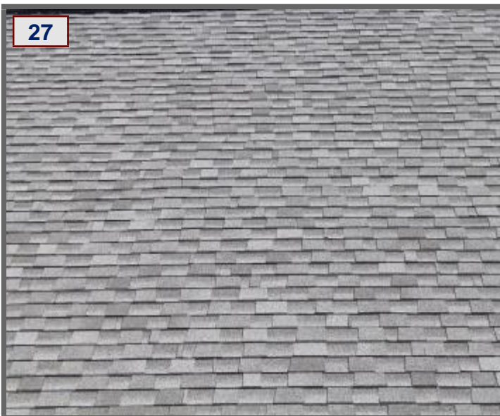
Shingles showing signs of weathering & age.
