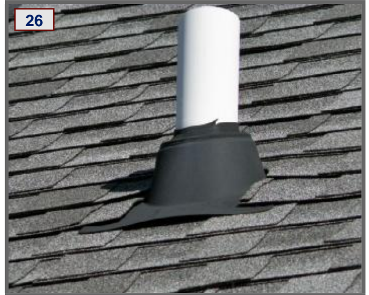
Shingles showing signs of weathering & age.
