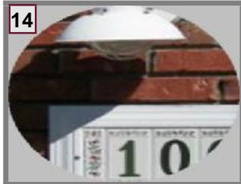
Front Light Bulb missing
